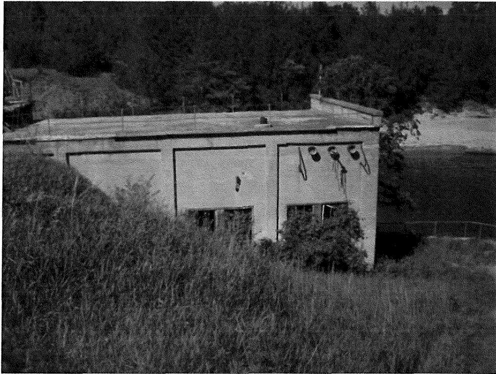
Photo 67 – Powerhouse south wall.
