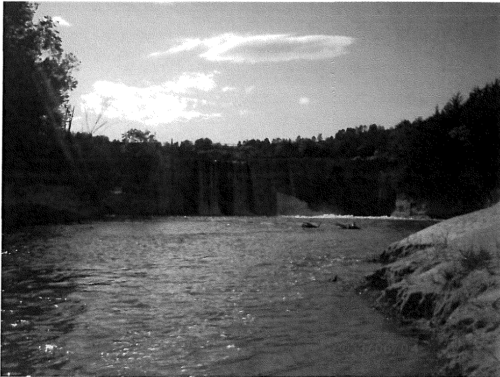
Photo 59 – McGowan Dam as seen from downstream.
