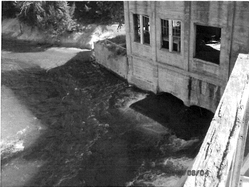
Photo 65 – McGowan Dam tailrace.
