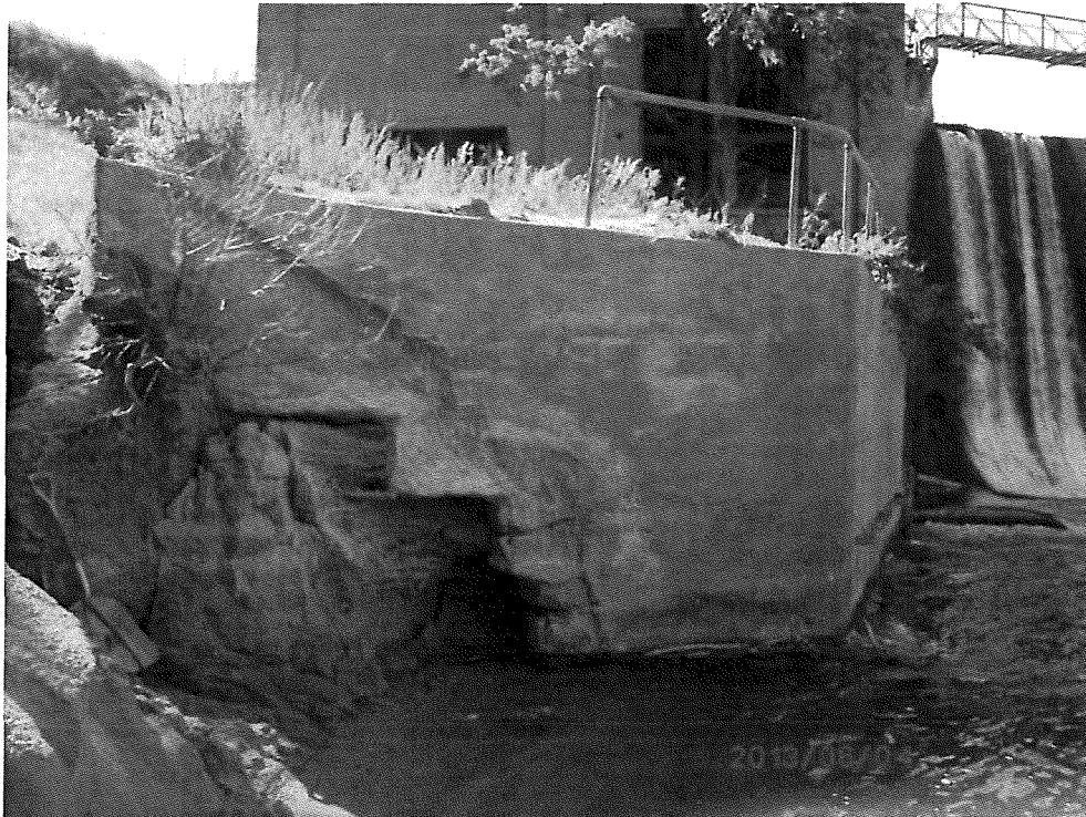
Photo 69 – Powerhouse trailing wall.
