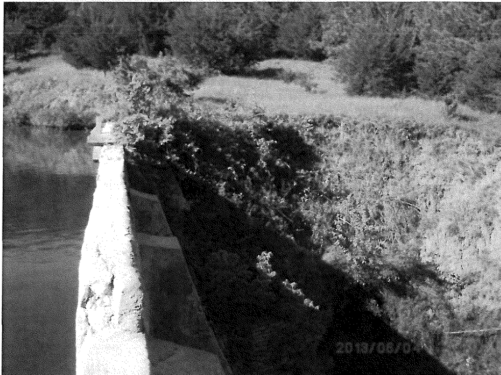
Photo 76 – Downstream of McGowan Dam.
