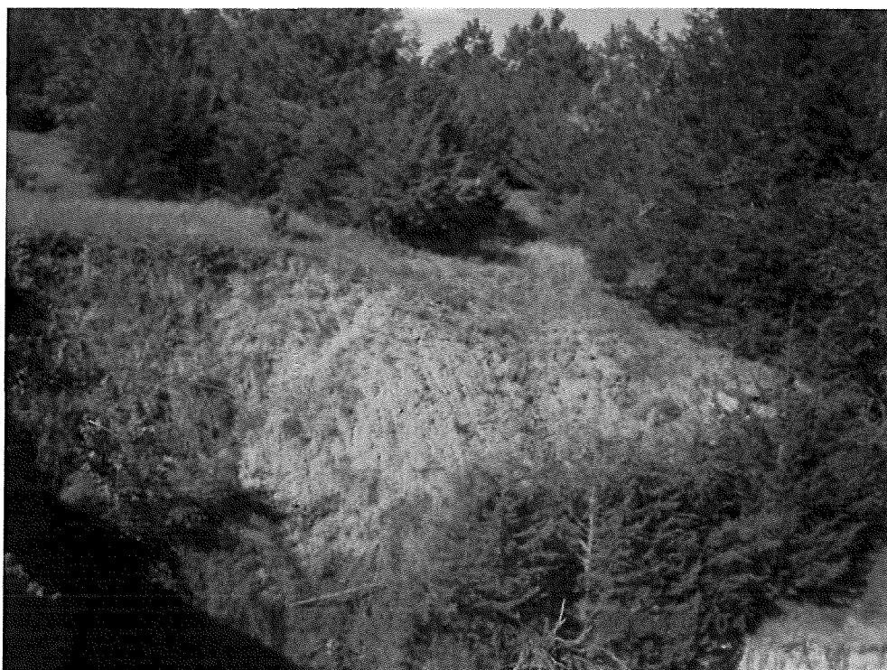
Photo 77 – Left abutment as looking downstream from McGowan Dam.
