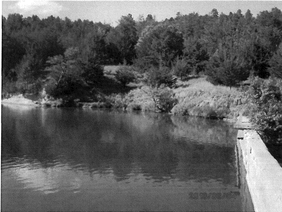
Photo 75 – McGowan Dam upstream left abutment.
