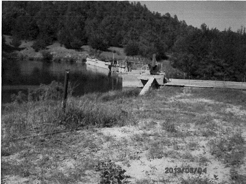
Photo 58 – McGowan Dam seen from upstream right abutment.
