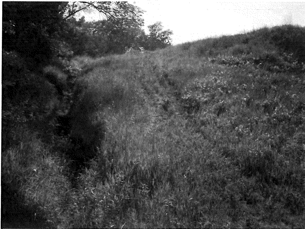
Photo 64 – Right abutment on downstream side.
