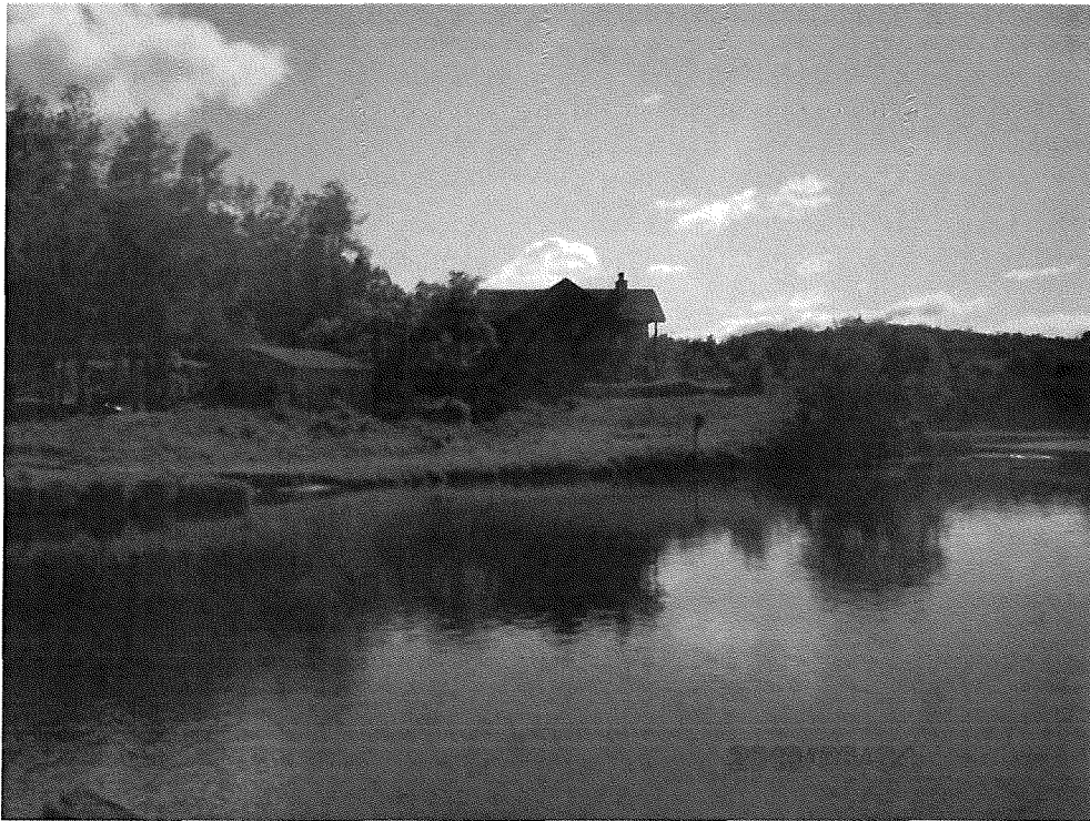
Photo 71 – Right banks of McGowan Reservoir as seen from dam.
