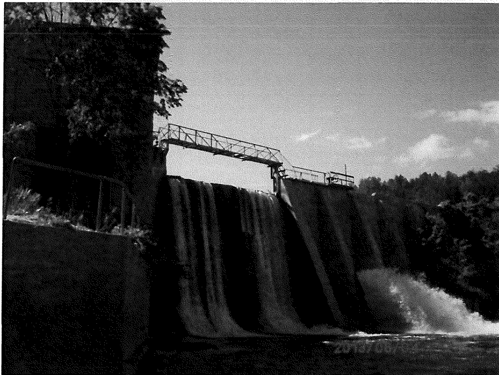
Photo 60 – McGowan Dam spillway and base discharge.
